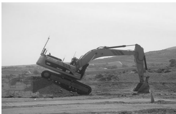
Fig.11 Operator action test in slope construction
