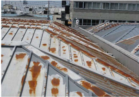
Before coating at rust surface
