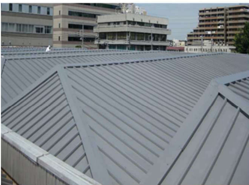
After bufferCoat10 coating
