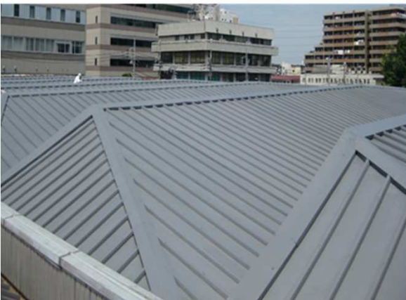
After bufferCoat10 coating
