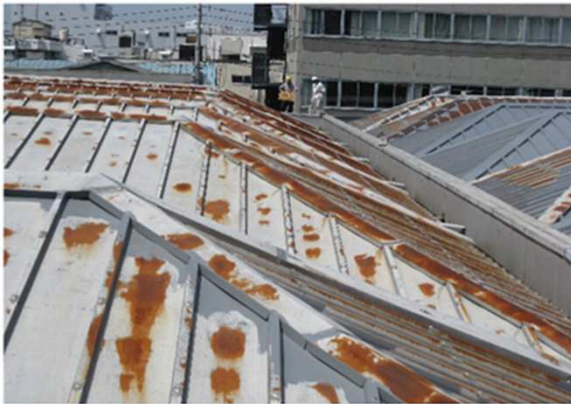
Before coating at rust surface
